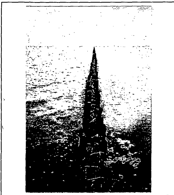
Fig. 4.4: Wave reduction by a brushwood groyne.
