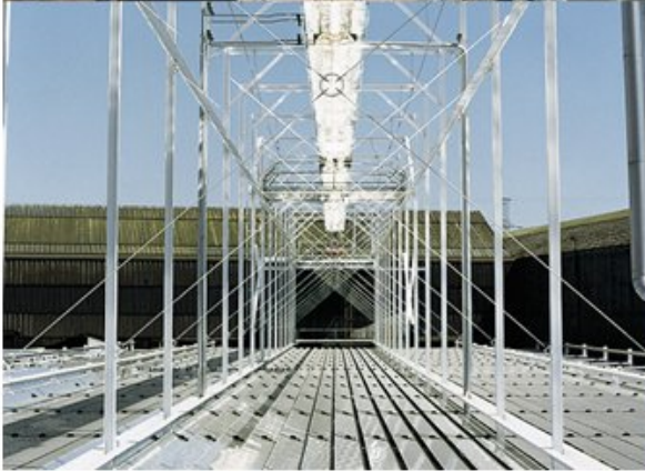
linear Fresnel (Solarmundo)
