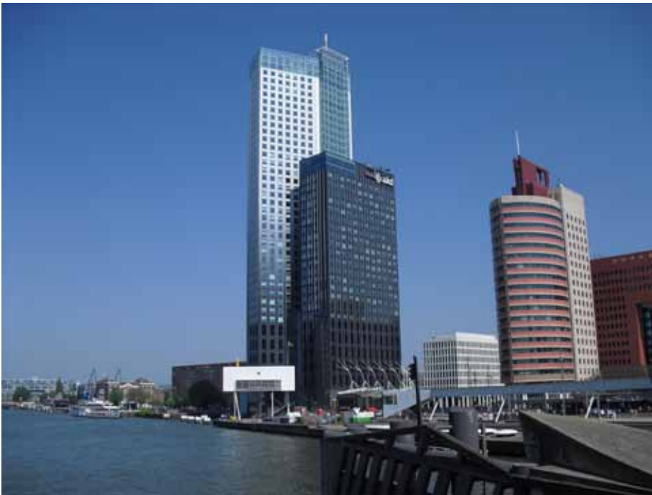
Photo 4 The Maas tower in Rotterdam, Netherlands. The new 160 m office building uses water from the Meuse River in combination with underground heat and cold storage as sources for its climate control systems thereby reducing its CO 2 footprint.
