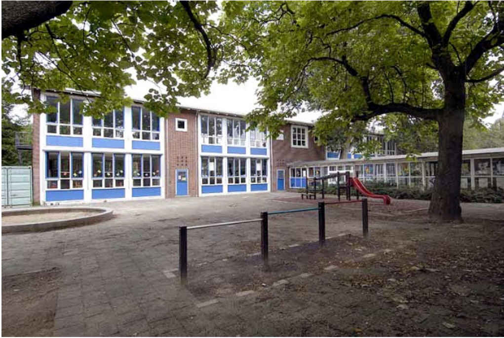
H-school, Amsterdam, 1954-1960 Architect: J. Leupen Bron: Kempinga en Wessel (2013)
