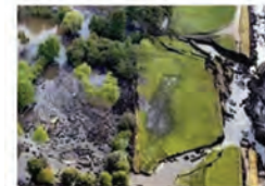
Levee breakthrough (drought)
