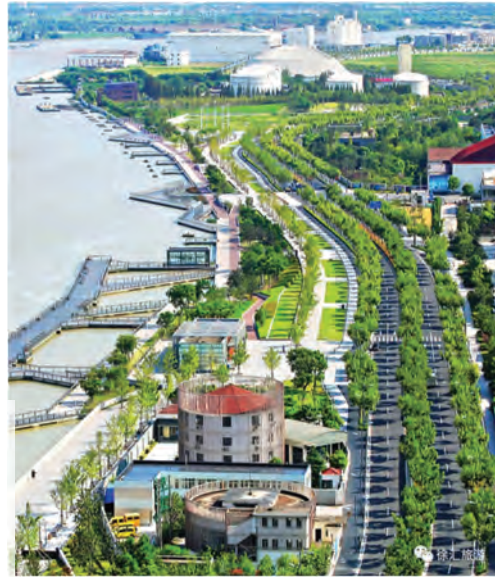
Shanghai West Bank Urban Waterfront Park Reconstructed from Wharf Area
