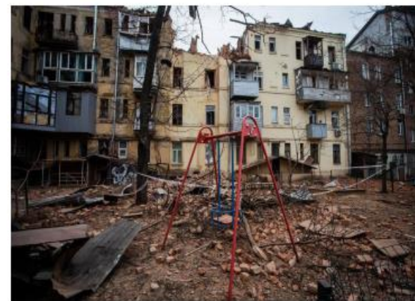
Building damaged by a russian S-300 missile in Kharkiv
