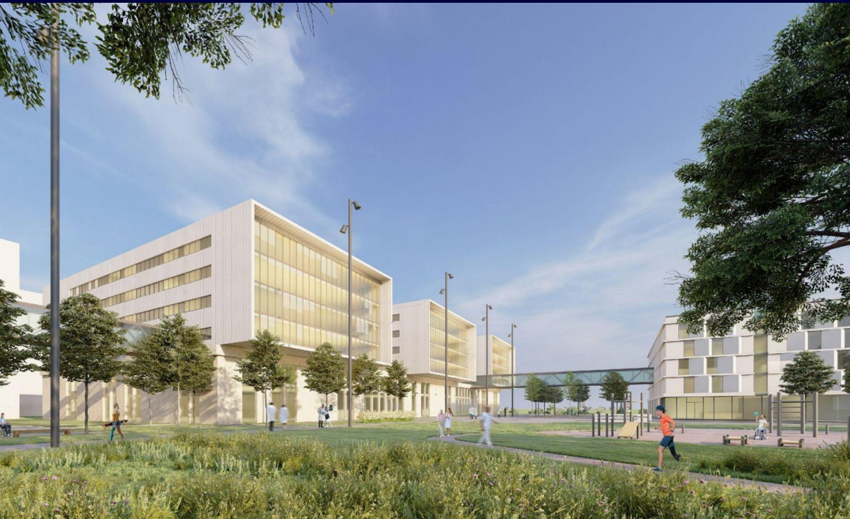
New buildings for surgery and rehabilitation
